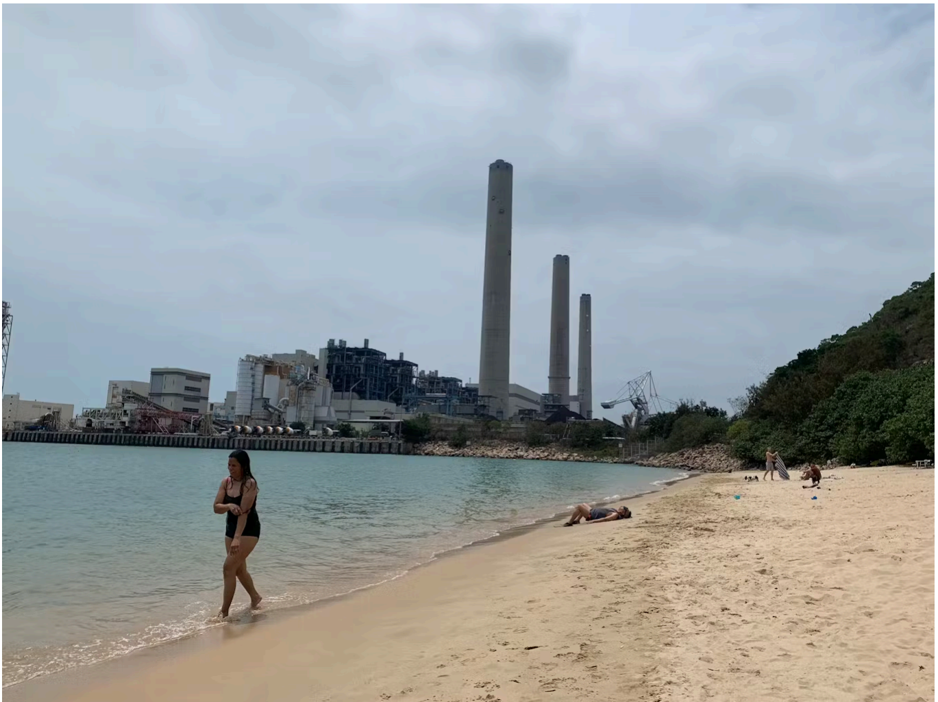
Power Station Beach by day. Beach-goers tend to position their towels away from the power station so that it isn't in view, says former resident Mark Counsell. Image: Robin Hicks / Eco-Business
