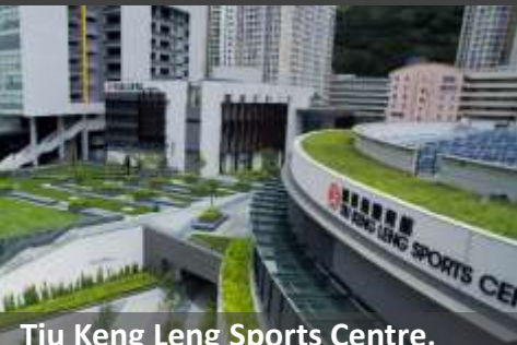
Tiu Keng Leng Sports Centre, Public Library and District Open Space
